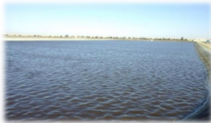
Figure 14: Lagune de finition.
