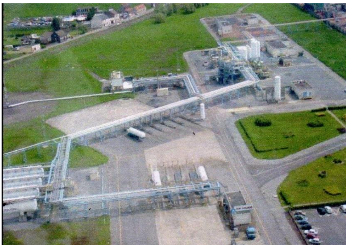
Figure 5.15 Air Liquide site in Waziers
