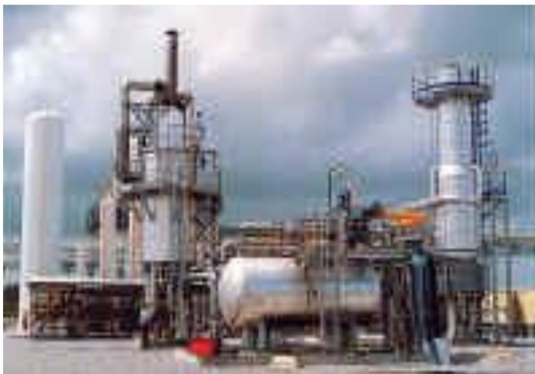
Figure 5.16 Hydrogen liquefier at the Kourou aerospace launch site
