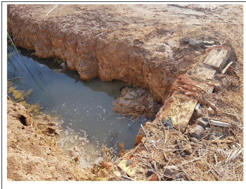
Figure II.33 : Milieu agressif (tranché de drainage)
