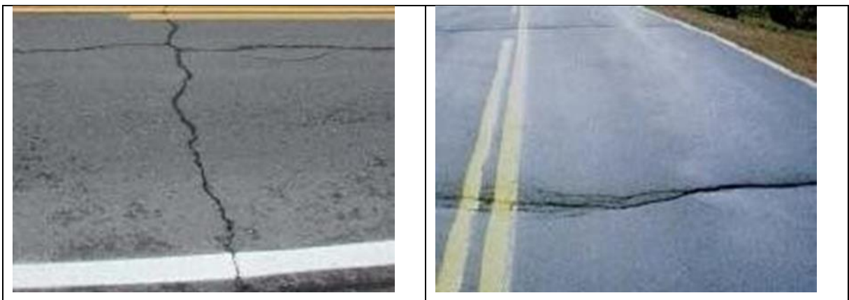
Figure 2.3. Fissures transversales
