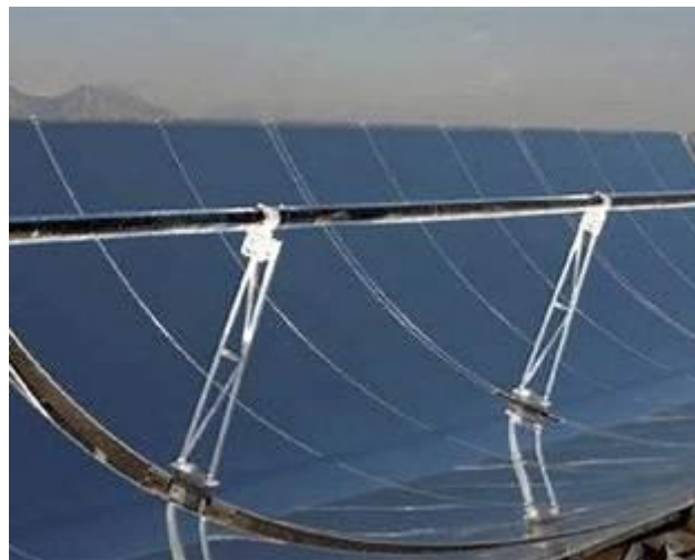
Figure I 3: Parabolic Trough Reflector. (NREL / SkyFuel)
