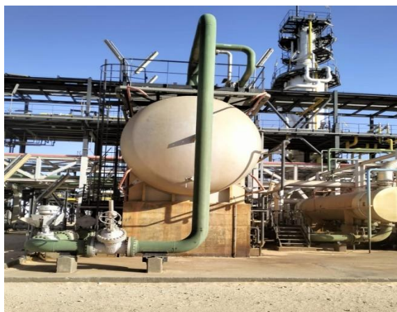
Figure I-7: The three-phase separator
