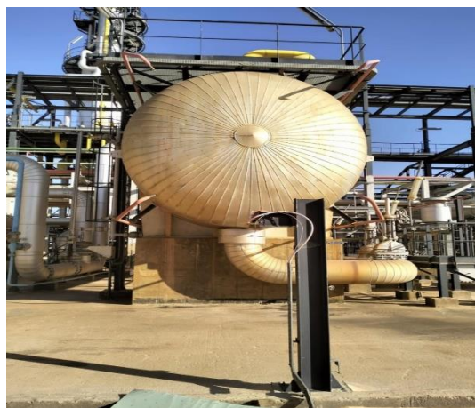
Figure I-8: The two-phase separator
