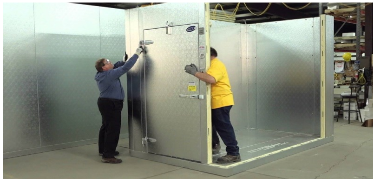
Figure III. 4: Installing of cold room
