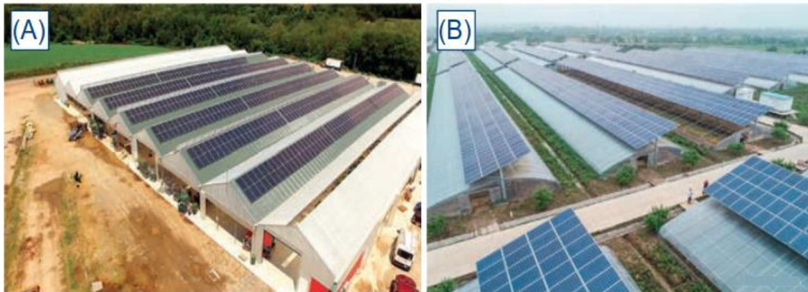
Figure I.17: (A) Solar PV panels mounted as a part of the roofs in commercial greenhouses implemented at Prides Corner Farms, and (B) The PV systems installed close to the greenhouses in Hongxingqiao Town, Changxing County, in east China's Zhejiang Province
