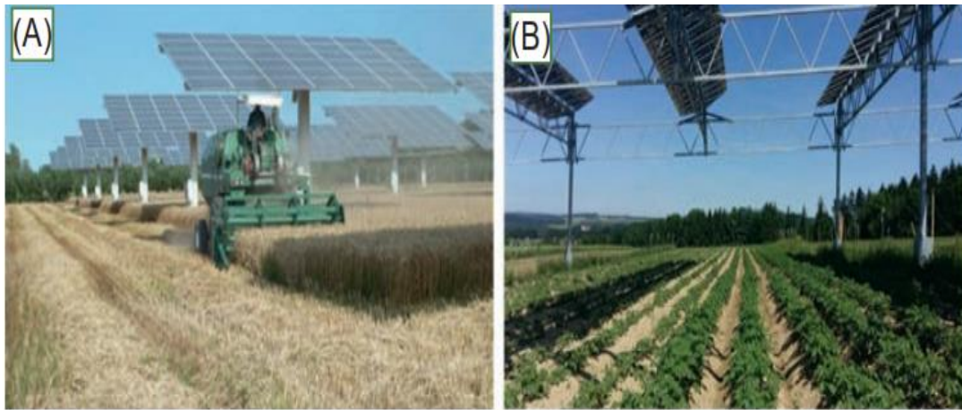
Figure I.12: (A) APV system installed in Italy, and (B) APV facility installed above the potato farm (RESOLA project), Heggelbach, Germany
