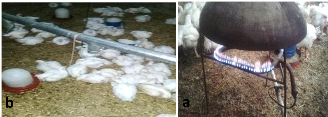
Fig. II.16. Photos of heating system components inside the shed: a) Open direct fire flame, b) Airdistribution perforated metal tube.[57]
