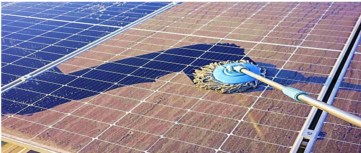
Figure (I.9): Cleaning process of removing accumulated dust from the photovoltaic panel surface.
