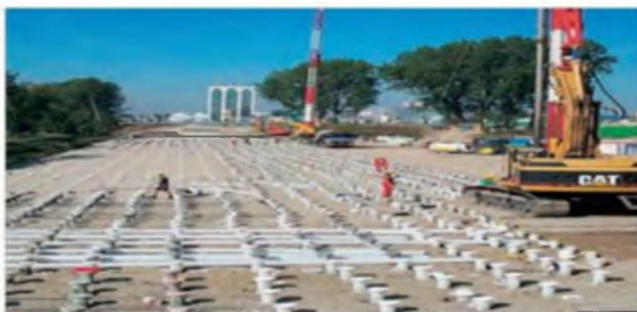
Figure 1.23. Principe Installation des drains.
