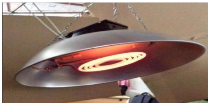
Fig II.10: Electric heaters in poultry houses [40].
