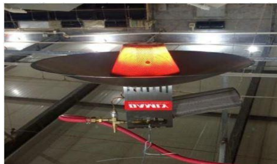
Fig II.17. Schematic diagram illustrating the operation of the heating radiator used in the poultry house [73].
