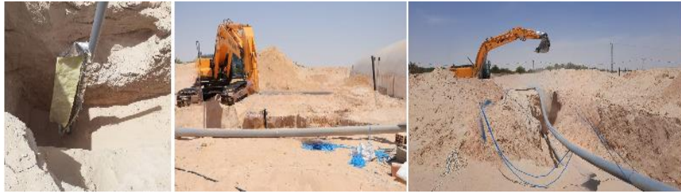
Figure II.9 Installing a geothermal system in an area (Reguiba-El Oued)
