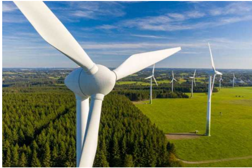
Figure (I.7). Wind Turbine.
