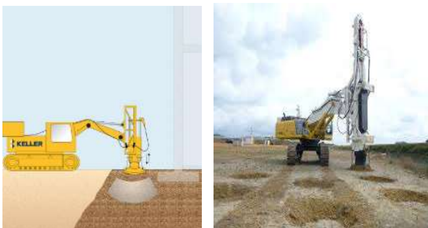
Figure I-16. Le Rapid Impact Compaction
