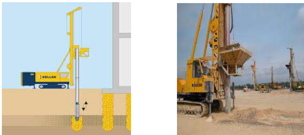
Figure I-11. colonnes ballastees
