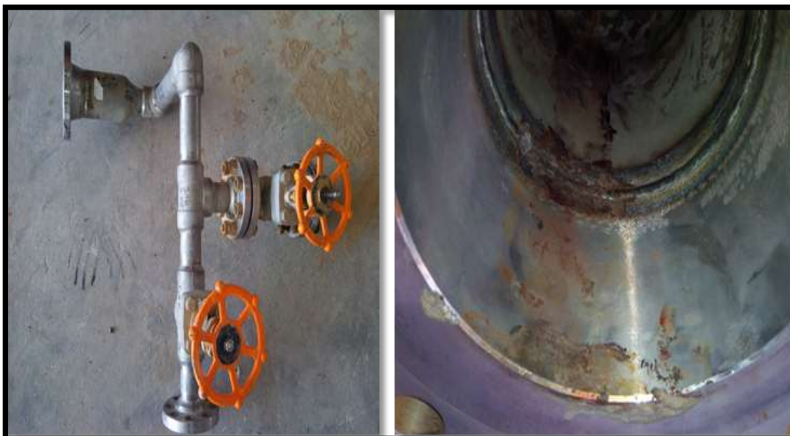
Figure III.3. Percement sortie filtre (CPF)
