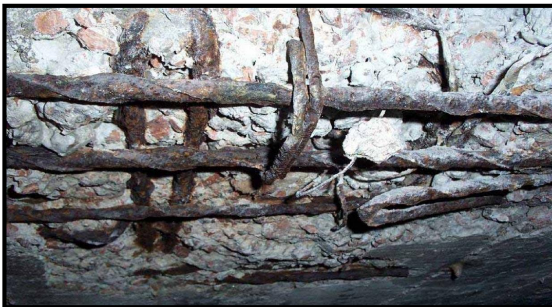
Figure 1.2: Erosion beton
