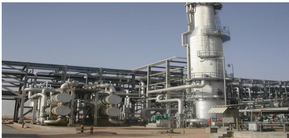
Figure II.14: La section stabilisation haute pression.
