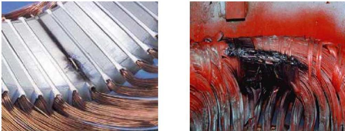
Fig. I.6. Damage caused by a IM's stator short-circuit faults.
