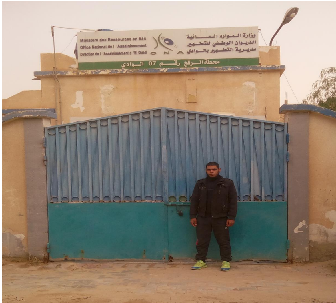
Photo II-4: Station de relevage
