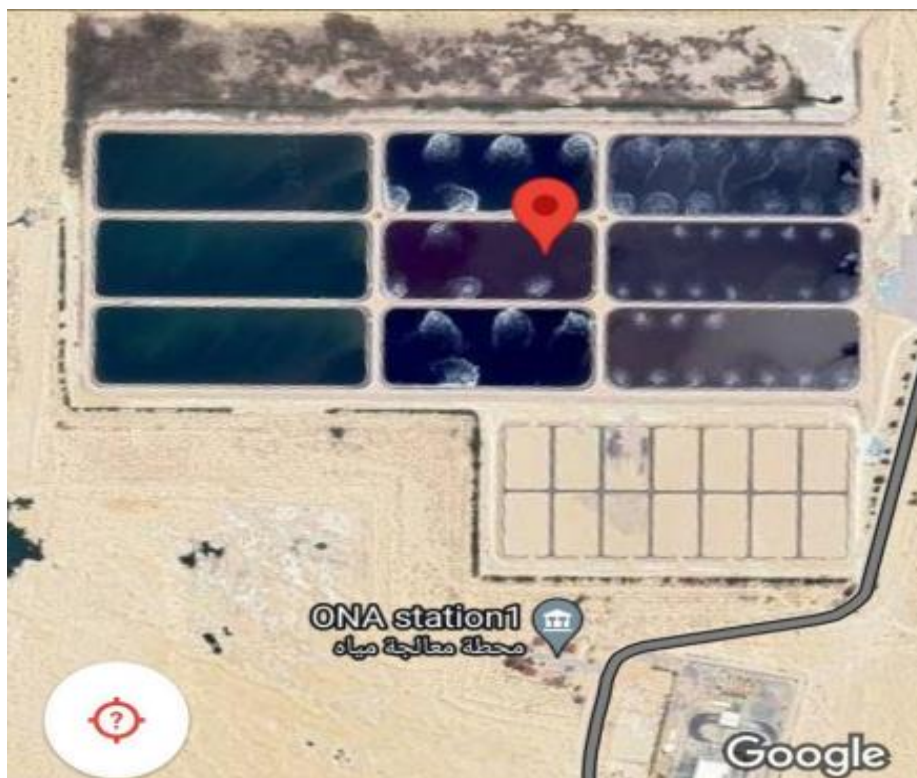
Figure 12 : Station d'épuration des eaux usées Kouinine – El'Oued (Google map, consule 10/06/2023).
