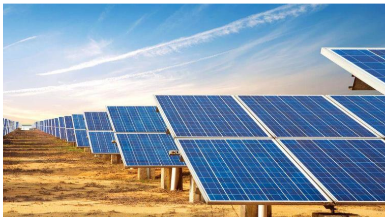
Figure I.2 Champ photovoltaïque fixe. [74]
