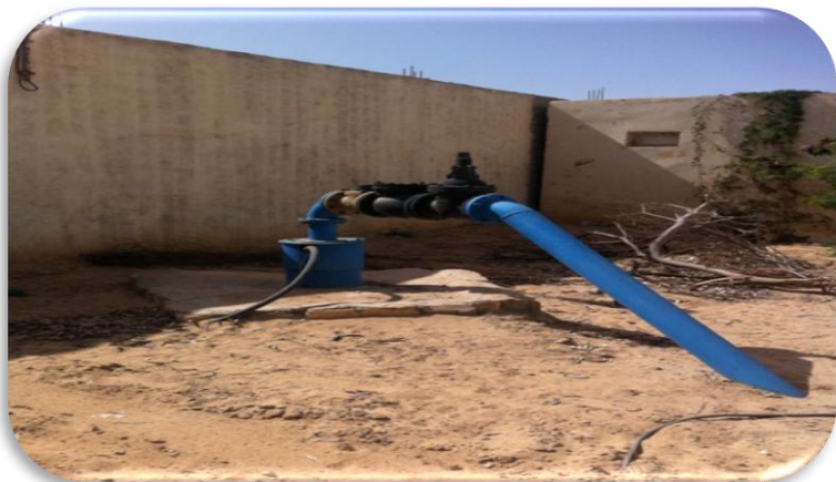
Figure II.1 : photo du forage 300 logs2014
