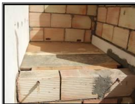
Fig.6. Realization of the wood board ceiling
