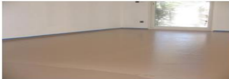
Figure I 4 Les chapes fluides chape ciment[3] .
