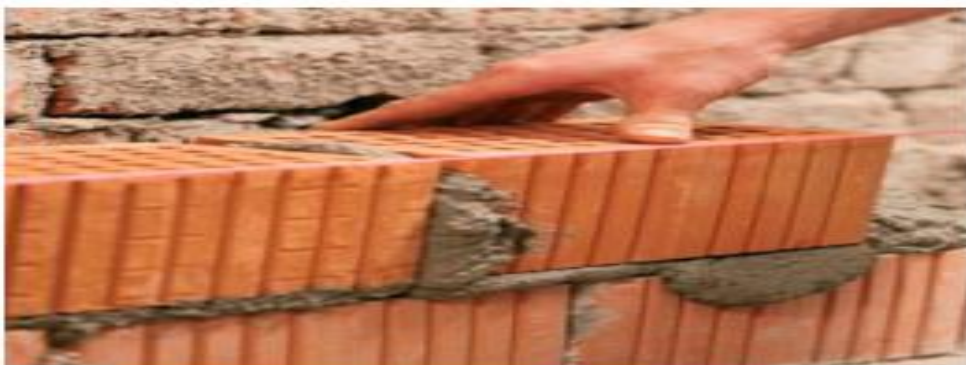
Figure I 2: pose de mortier de hourdage[3].
