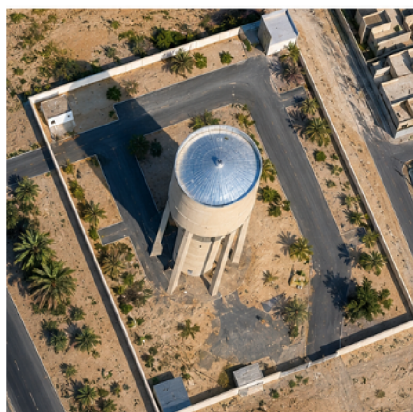
Figure 4.2: Aerial view of the Château d'eau (elevated storage reservoir) supplying the University Hamma Lakhdar campus distribution network, El Oued.
