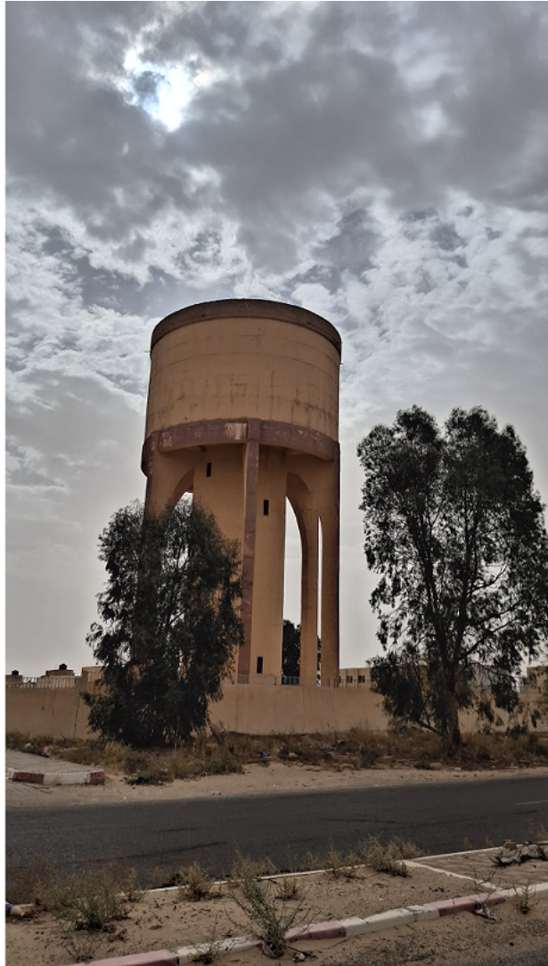
Figure 4.1: Photographic overview of the University Hub Pumping Station installation site, University Hamma Lakhdar, El Oued.
