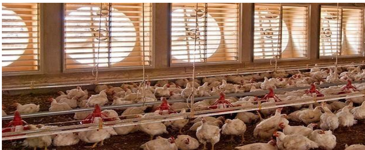
Figure II. 6: Ventilation in poultry houses.
