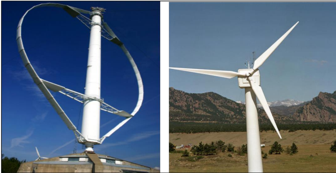
Figure I. 8: Vertical Axis Wind Turbine (VAWT) Figure I. 9: Horizontal Axis Wind Turbine (HAWT) I.4.2.1. Horizontal wind turbine types:
