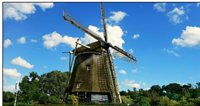
Figure I. 3: Old windmill (Netherland)
