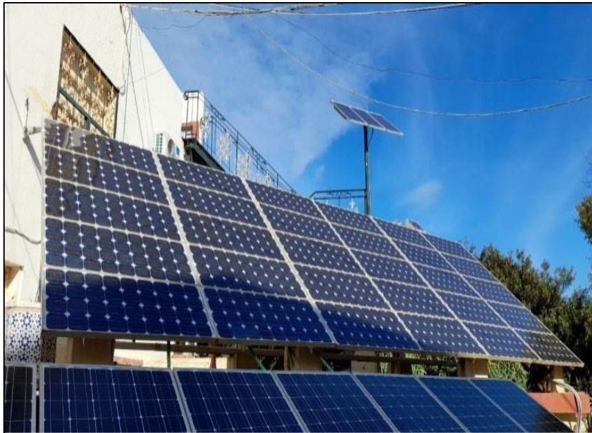
Figure 2.27. Building shading on the panels
