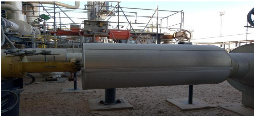
Figure III.9: The turbo expansion of the LPG2 unit[34].
