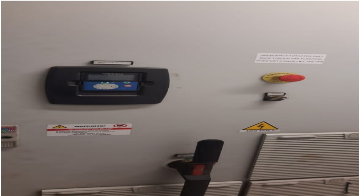
Figure II. 9: The Variable Frequency Drive (VFD).
