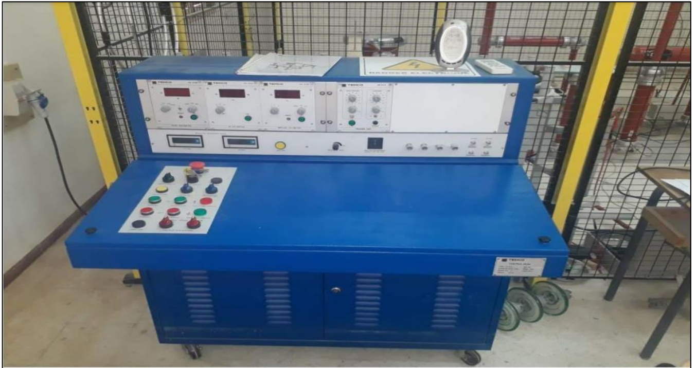
Figure III.2. Photo of the control panel in the high voltage laboratory at the University of El Oued.
