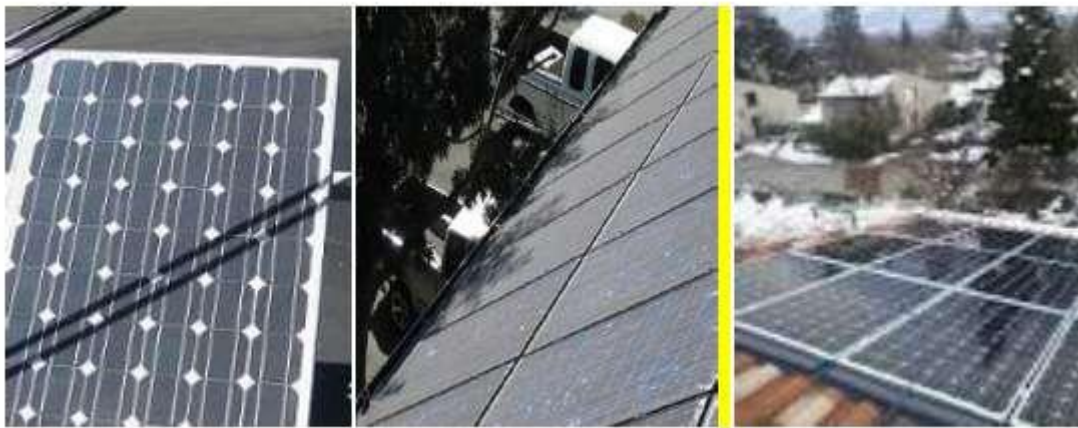
Figure (III.12): Partial Shading Fault Diagram
