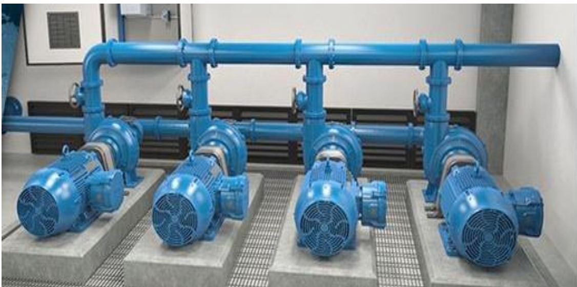
Figure I.4 : Station de rejet [2]
