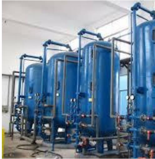
Figure I.2 Station de filtre à sable [2]
