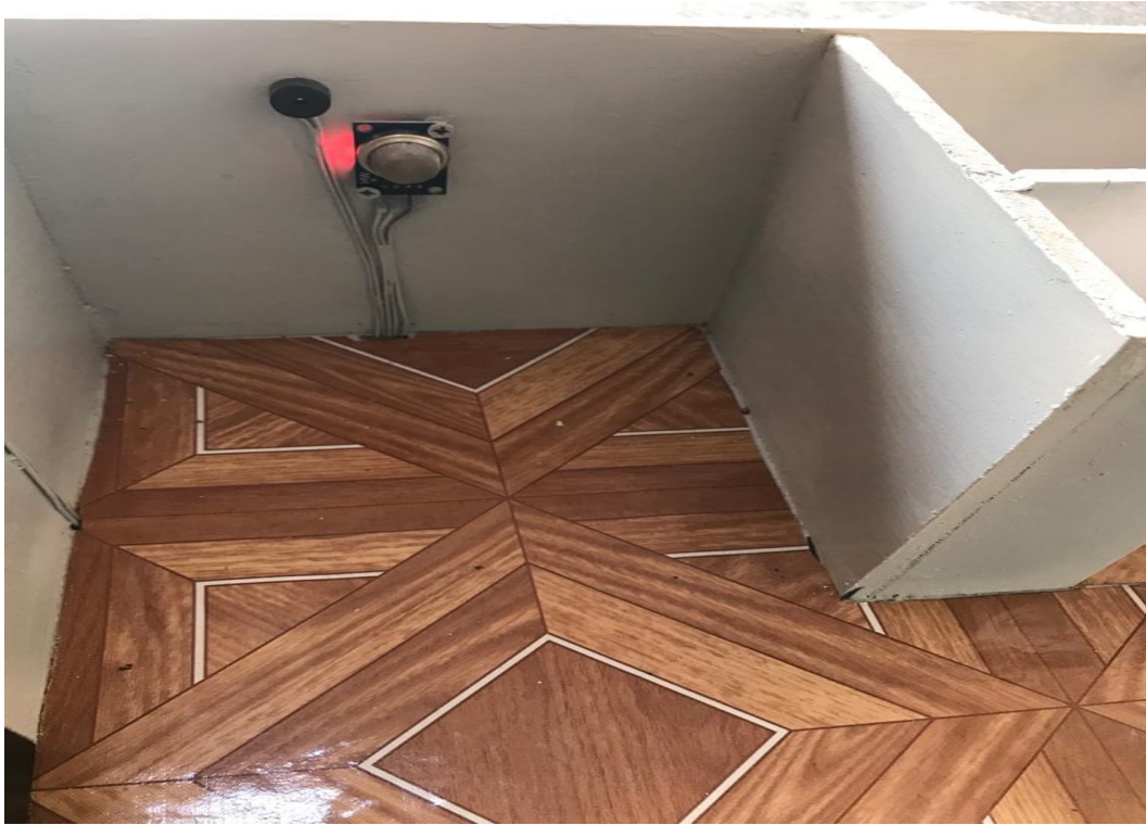
Figure III.27 : installing and testing gas sensor (MQ2)
