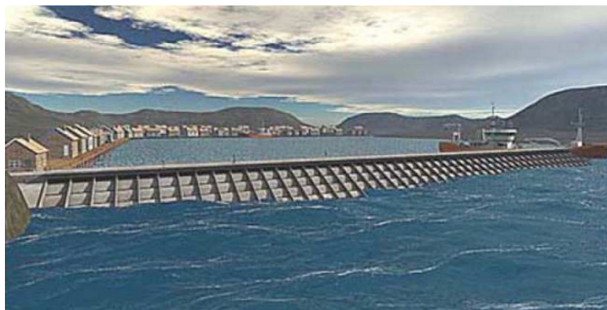
Figure II.21 Système Seawave Slot-cone Generator
