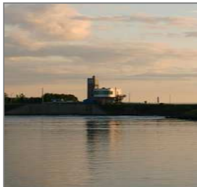
Figure II.4: Usine marémotrice Annapolis Royal, Nova Scotia, Canada[14]
