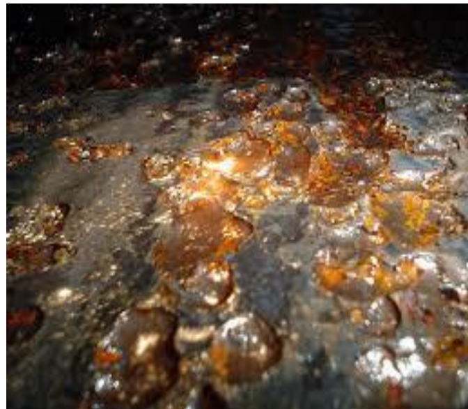
Figure 1.4: Metal affected by pitting corrosion.
