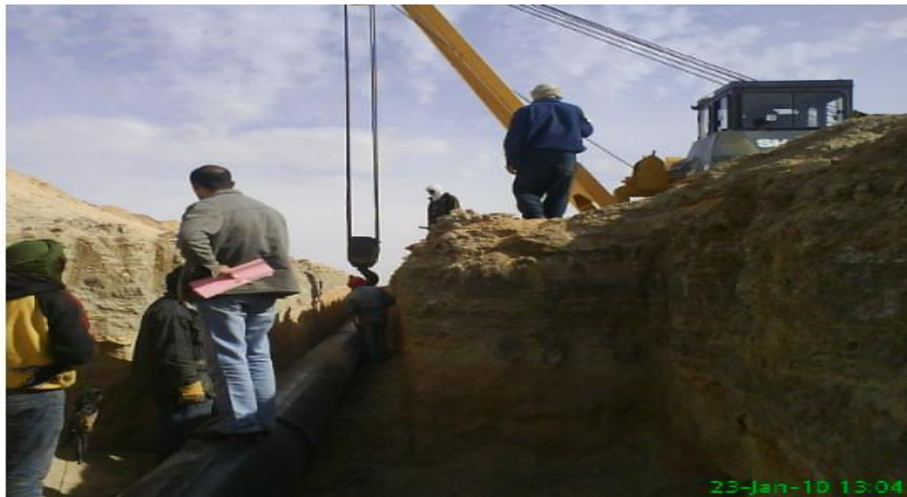
Figure III.9 : Raccordements (Gazoduc Djamaa-Touggourt)
