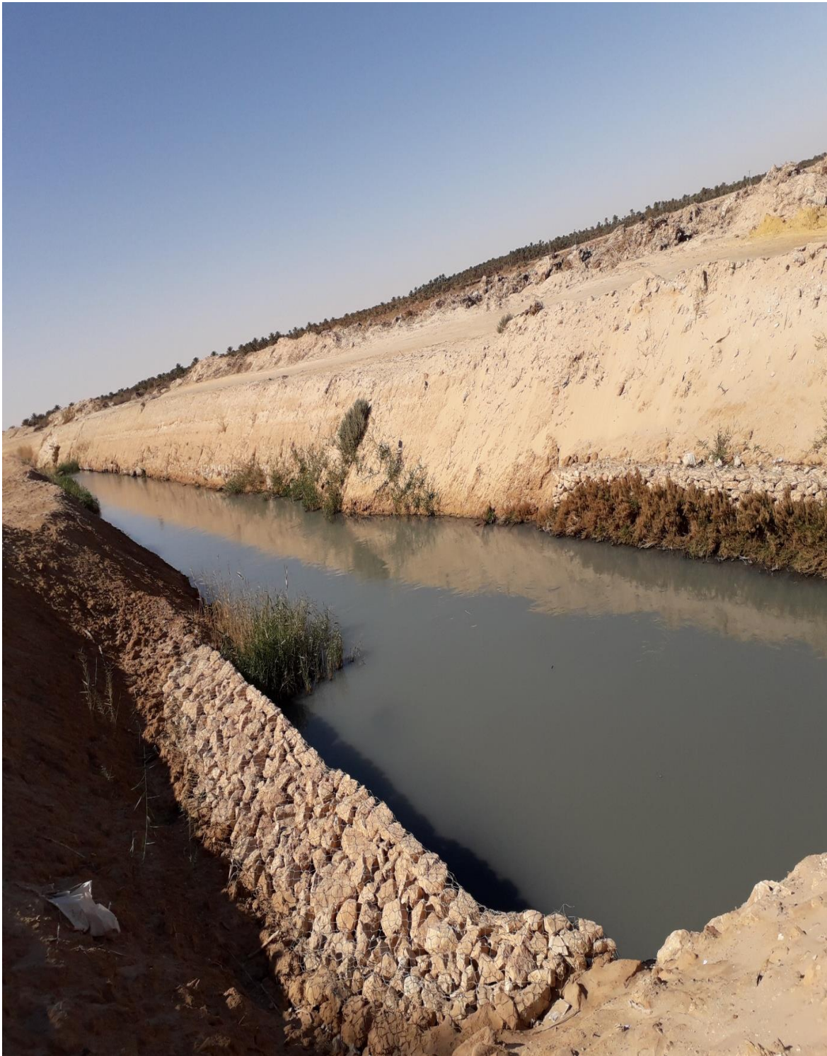
Photo (III.3.) : station Kardache (Bouaichi et B.A.Allah2019)
