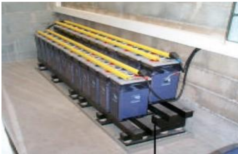
Figure II.9: Batteries d'accumulateurs
