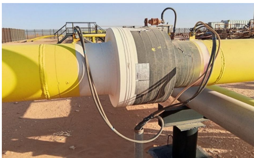
Figure 44 joints isolant monobloc 12''
