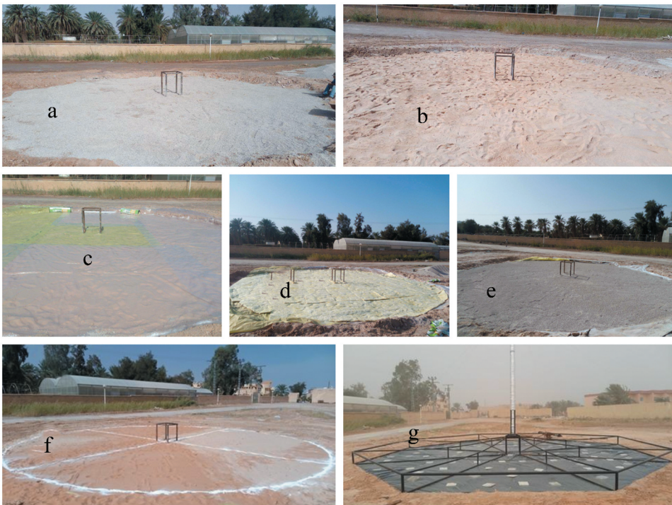
Figure 4. The thermal insulation steps of the solar chimney's ground (a: thick gravel, b: sand, c: plastic, d: Aluminum folio with glass wool, e: gravel, f: Sand, g: black plastic).
