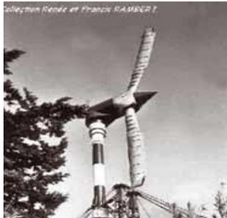
Figure I-10: 100 kW wind turbine from Grand Vent [11]
