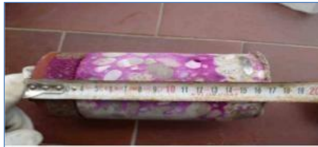
Figure II.7: Carbonatation sur carotte.
