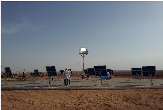
Fig. 6. Installation of the heliostats and test
