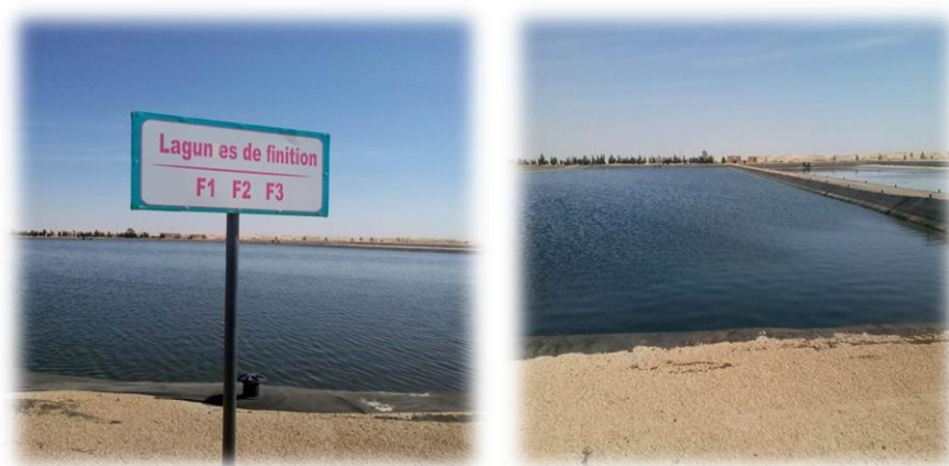
Figure 13: Lagune de finition.
