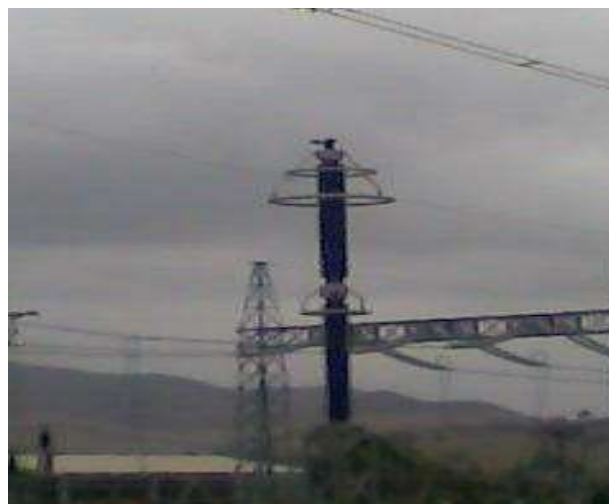
Figure 5.6 Parafoudre 400 KV [12]
