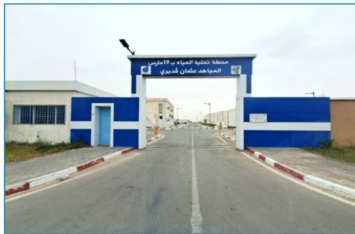
Figure 10: Photo of the entrance to the El-Oued desalination station.
