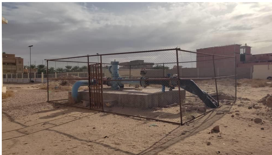
Image II.3: Le forage Albien de la station (ELCHOUHADA)
